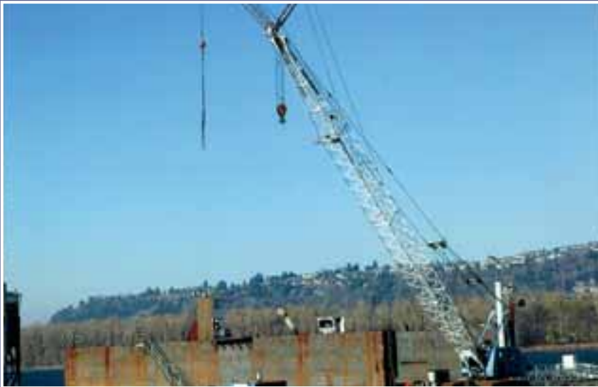
Manitowoc 3900 Vicon Crawler Crane
